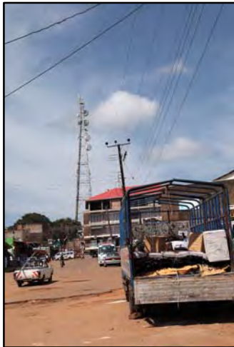
Well Constructed Cell Towers Appear Curiously Out-of-Place
