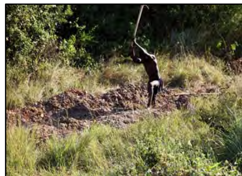
All Cable is being Installed using Manual Labor
