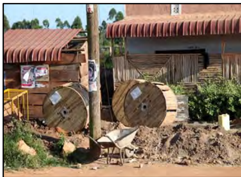
Fiber Optic Cable being Installed in Lukaya, Uganda
